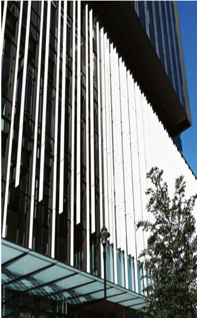
• New Headquarters Building, Seattle, USA
