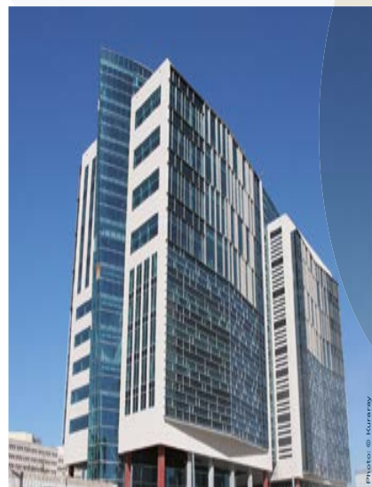
• Miami Courthouse, USA
