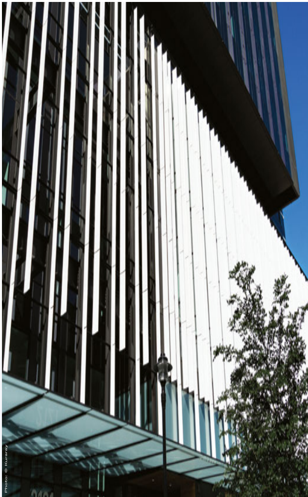
• New Headquarters Building, Seattle, USA
